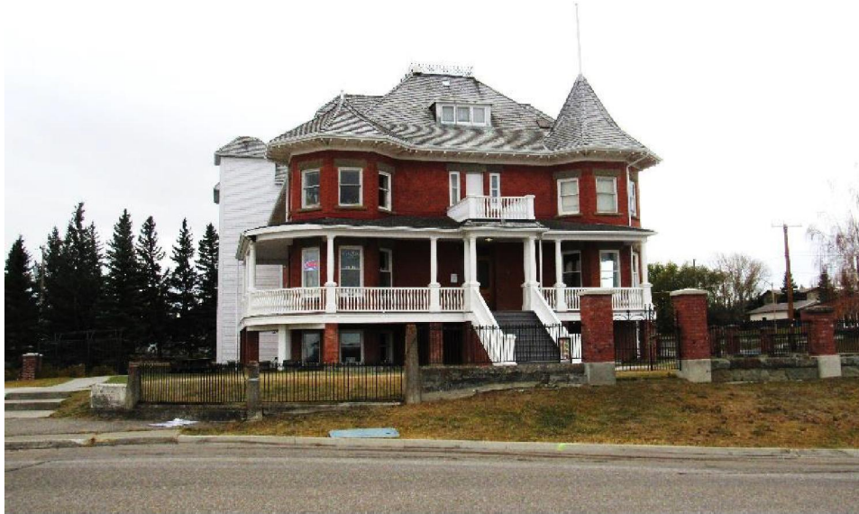
General view of the Site building.
